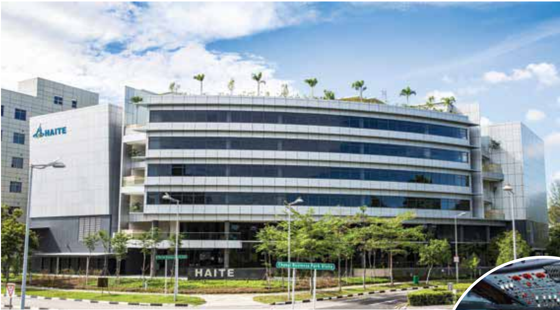
LEFT: Located in Changi Business Park, the HAITE Singapore Aviation Training Centre is a six-storey facility of over 21,000m 2
